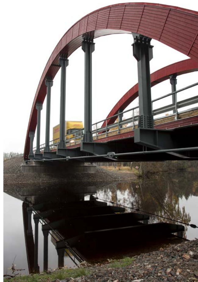
Bridge, Gislaved, Sweden.
