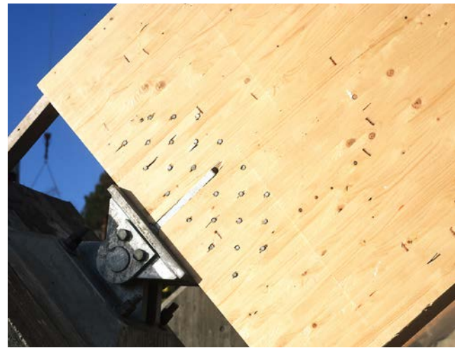
Arch with slotted-in steel plates and dowels, Kolmården zoo, Sweden.
