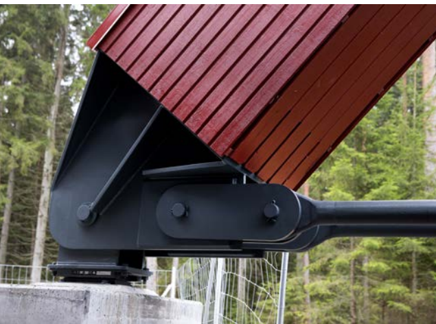
Bridge, Gislaved, Sweden.
