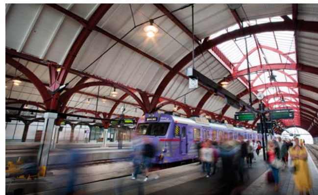
Malmö Central Railway Station main hall, built in 1923. This is one of the first great uses of glulam in Sweden. The station building is today in working order.
