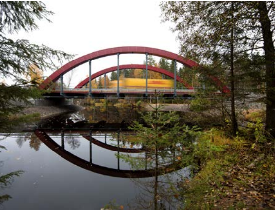
Bridge, Gislaved, Sweden.
