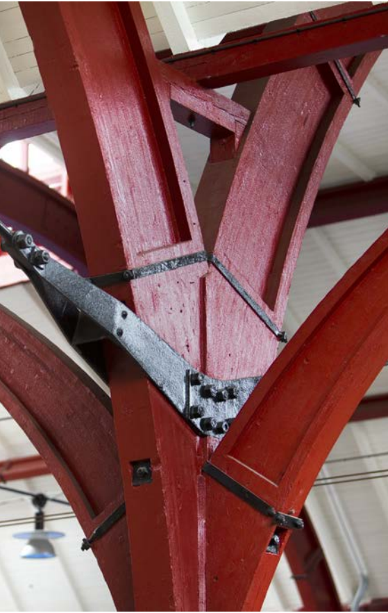
Detail of a joint at Malmö Central Station, Sweden.
