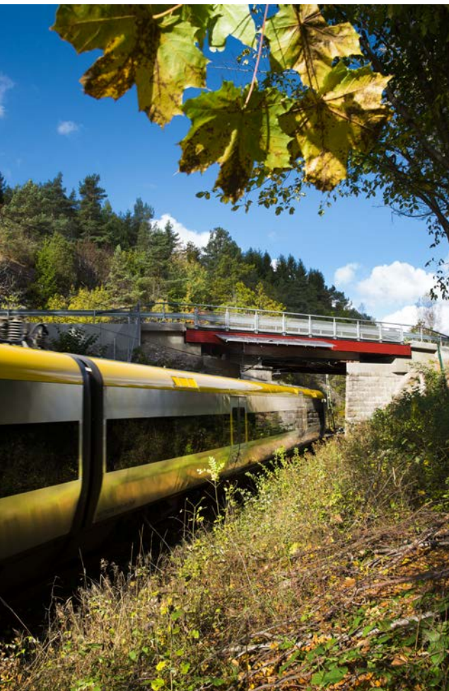
Railway bridge, Munkedal, Sweden.
