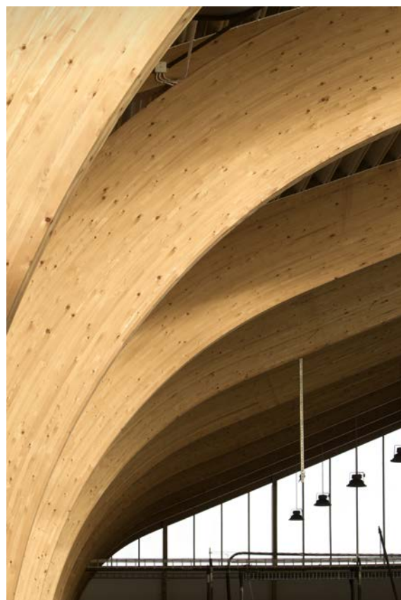
Three-pin glulam arches in cowshed.
