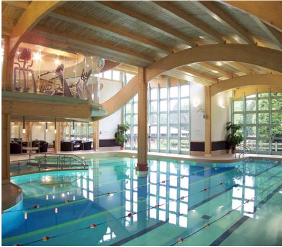
Bathing facilities with glulam frame.
