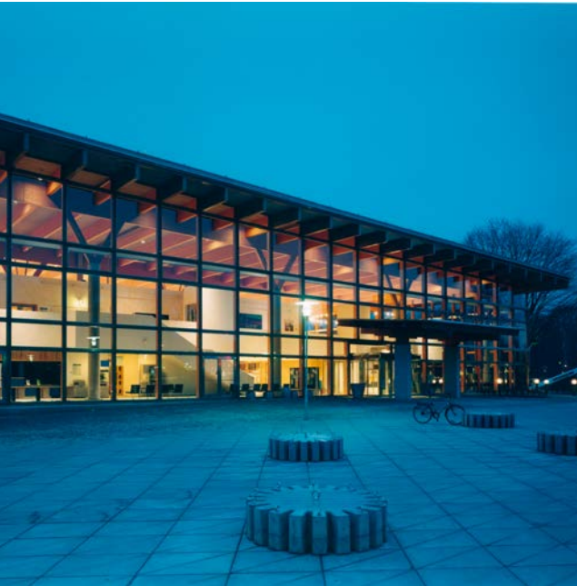
Library with glulam roof beams on concrete posts.
