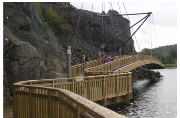
Footbridge made of timber and glulam, both pressure-treated.
