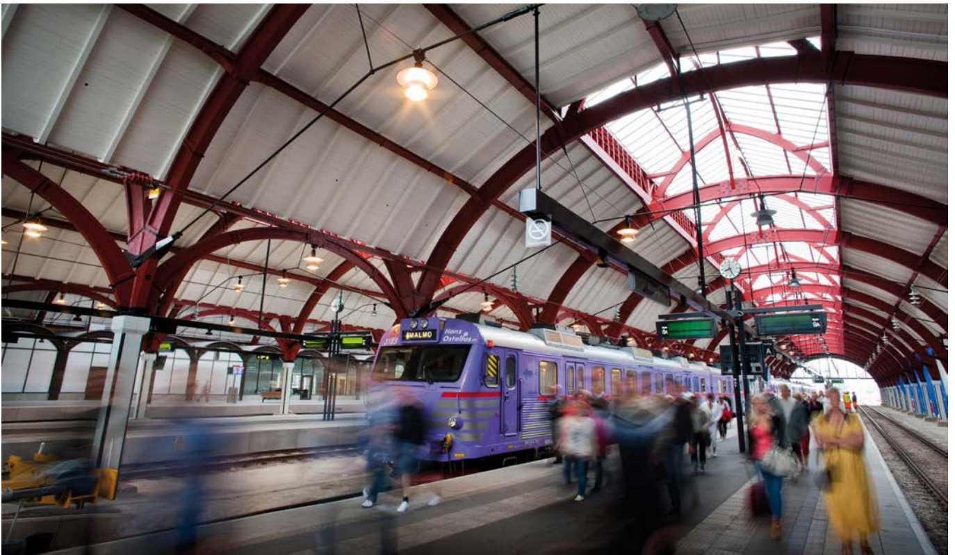
Malmö Central Railway Station main hall, built in 1923. This is one of the first great deliveries of glulam in Sweden. The station building is today in working order.
