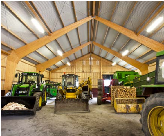
Machine shed made of three-pin frames with finger-jointed corners.
