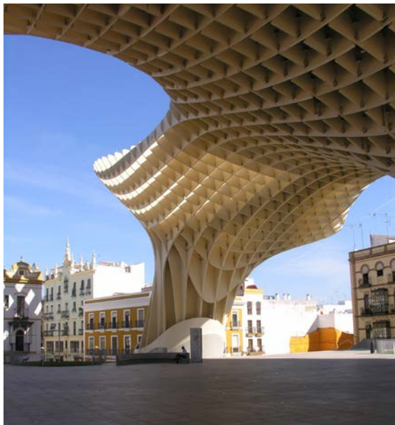
Metropol Parasol in Seville with protective polyurethane coating.
