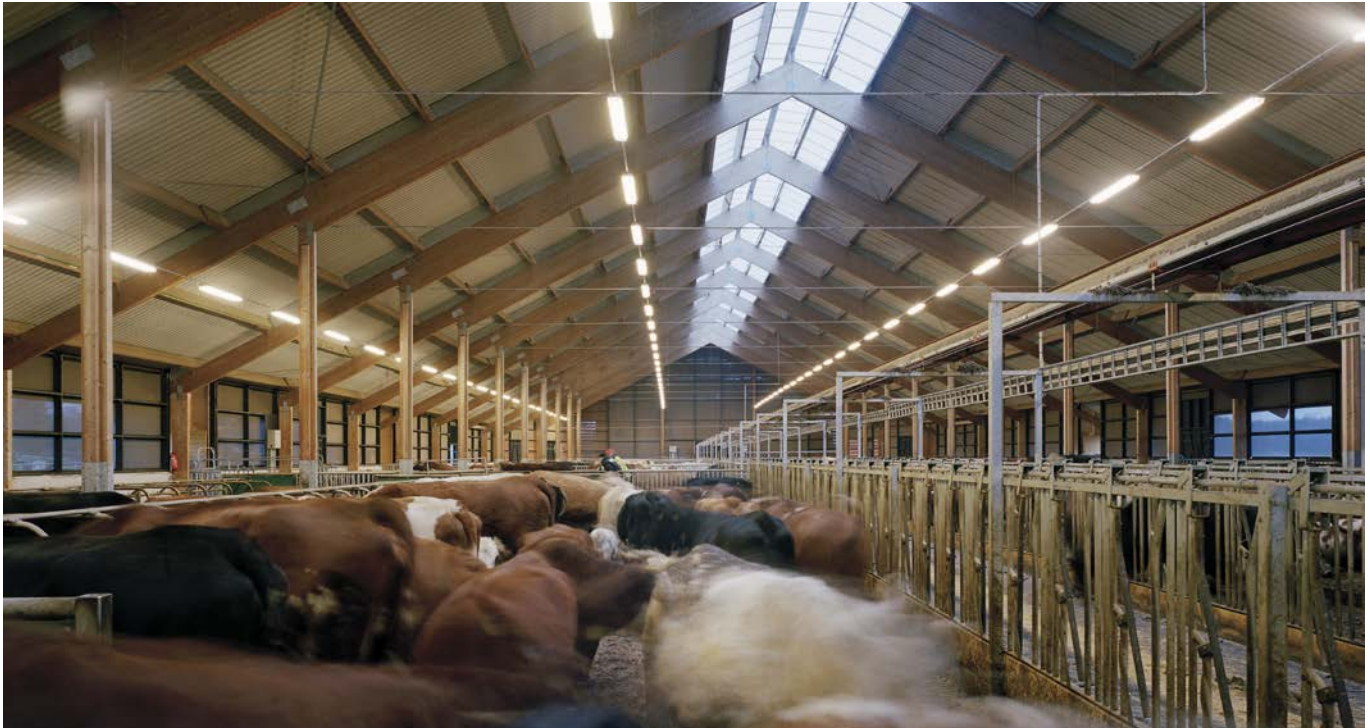
Cowshed with glulam frame.
