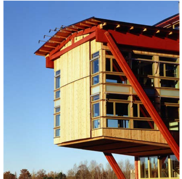
Office building with frame of glulam posts and beams. Composite floor structure in glulam and concrete.
