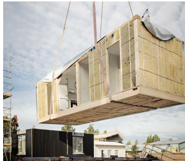
Volumetric units in CLT.
