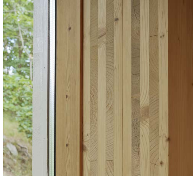
External wall made of CLT.
