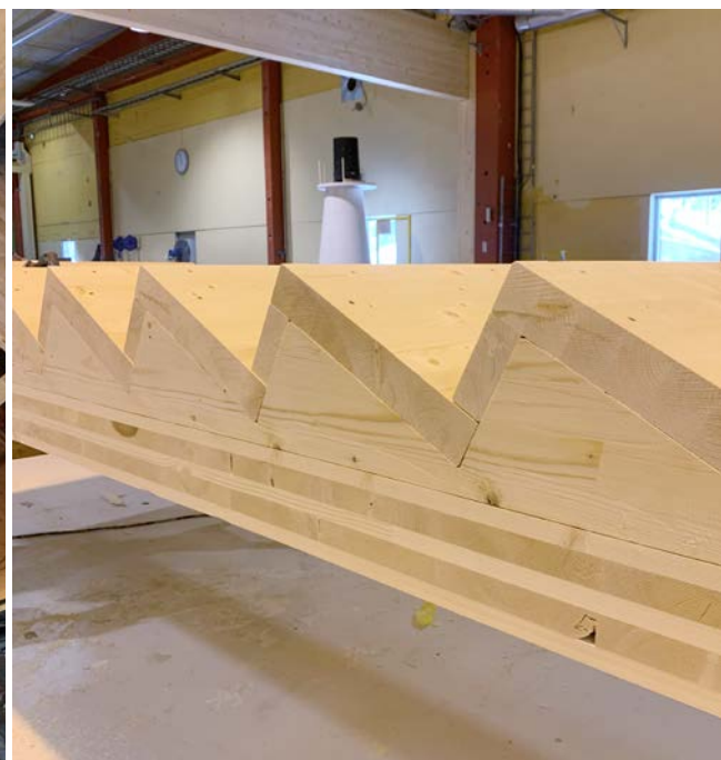
Stair carcass in CLT.
