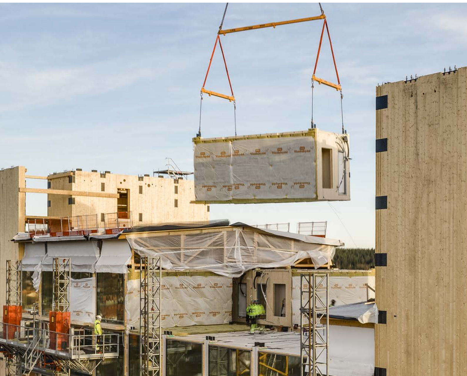
Volumetric units in CLT.
