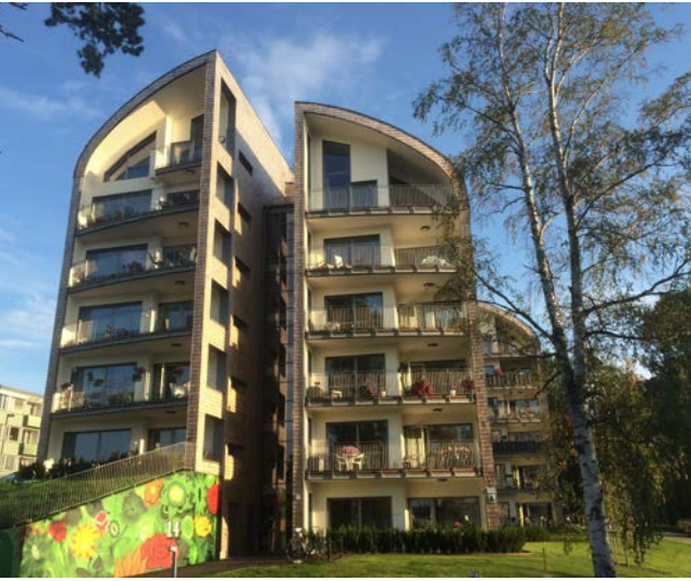
Six-storey apartment block with CLT frame.
