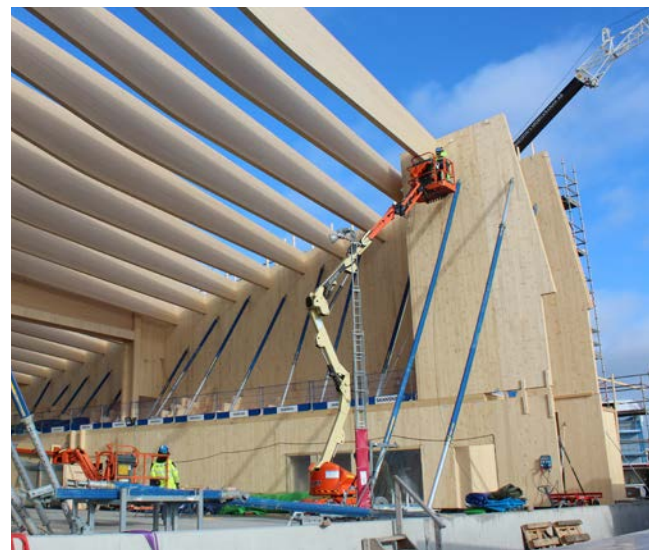
CLT and glulam working together.
