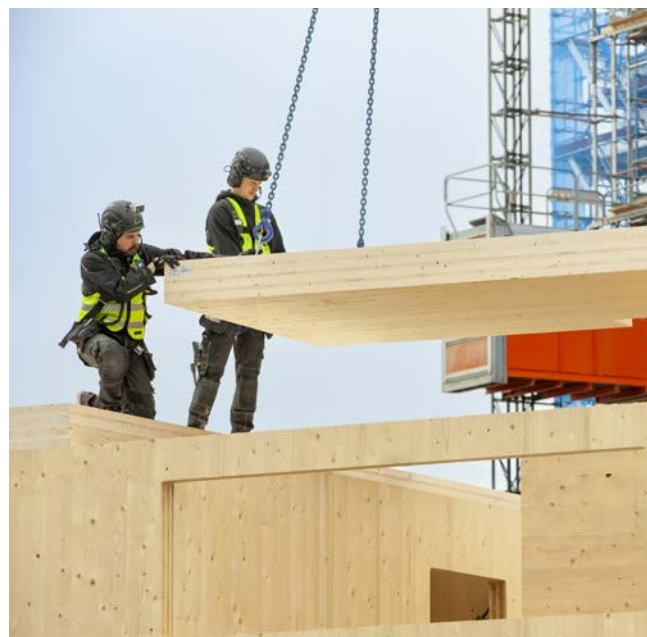
Installing a CLT floor slab.
