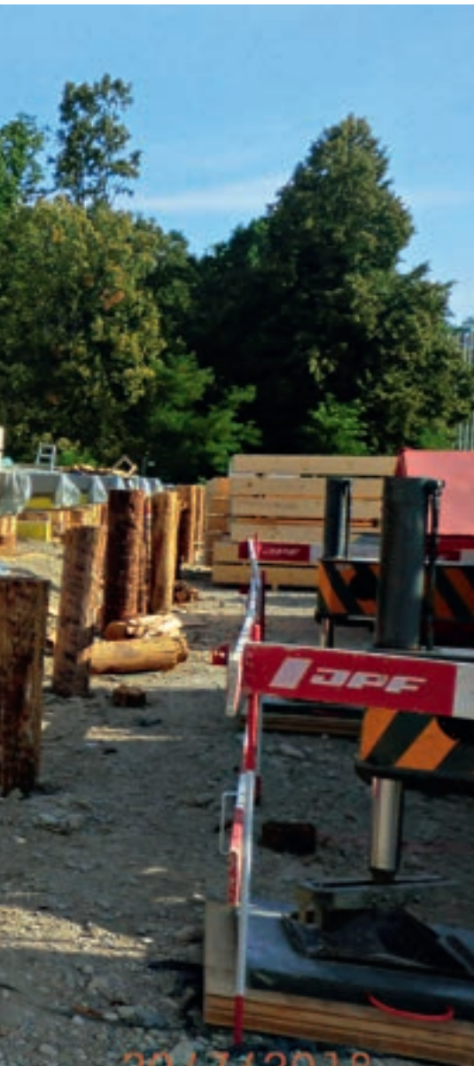
The foundations tend to account for a large part of a building's climate impact, but with debarked larch trees as piles, the footprint can be significantly reduced.
