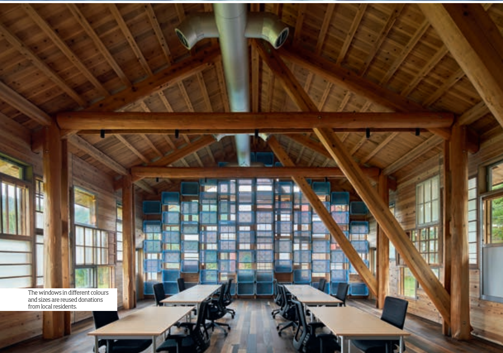
Between each pair of load-bearing posts sits a roughly sawn brace, secured in the roof ridge.
