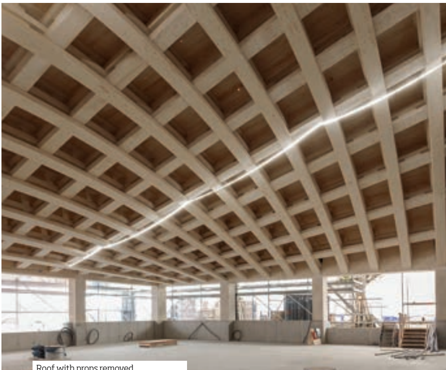
Roof with props removed.
