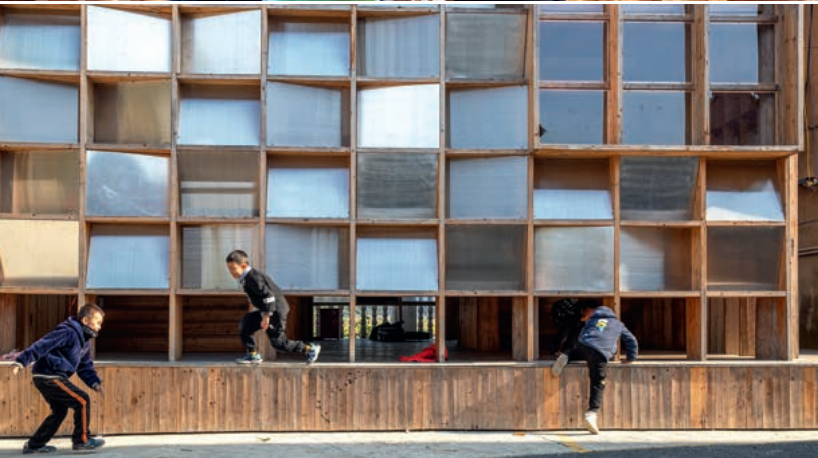
Polycarbonate sheets inserted into the gridded façade at different angles give a playful light effect.
