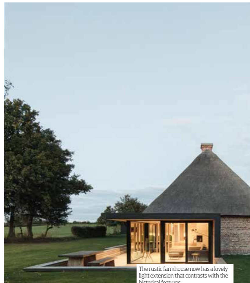
The pyramid shape reduces the wind load by shrinking the surface area of the roof. Light and air filter in through wooden screens.
