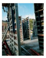
Spruce plywood is ideal for concrete formwork because of its strength and rigidity, and can be re-used several times if appropriate care is taken.
